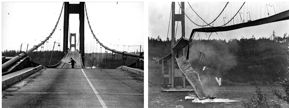
Figure 1.1.: Oscillations and collapse of the Tacoma Narrows Bridge [98].
