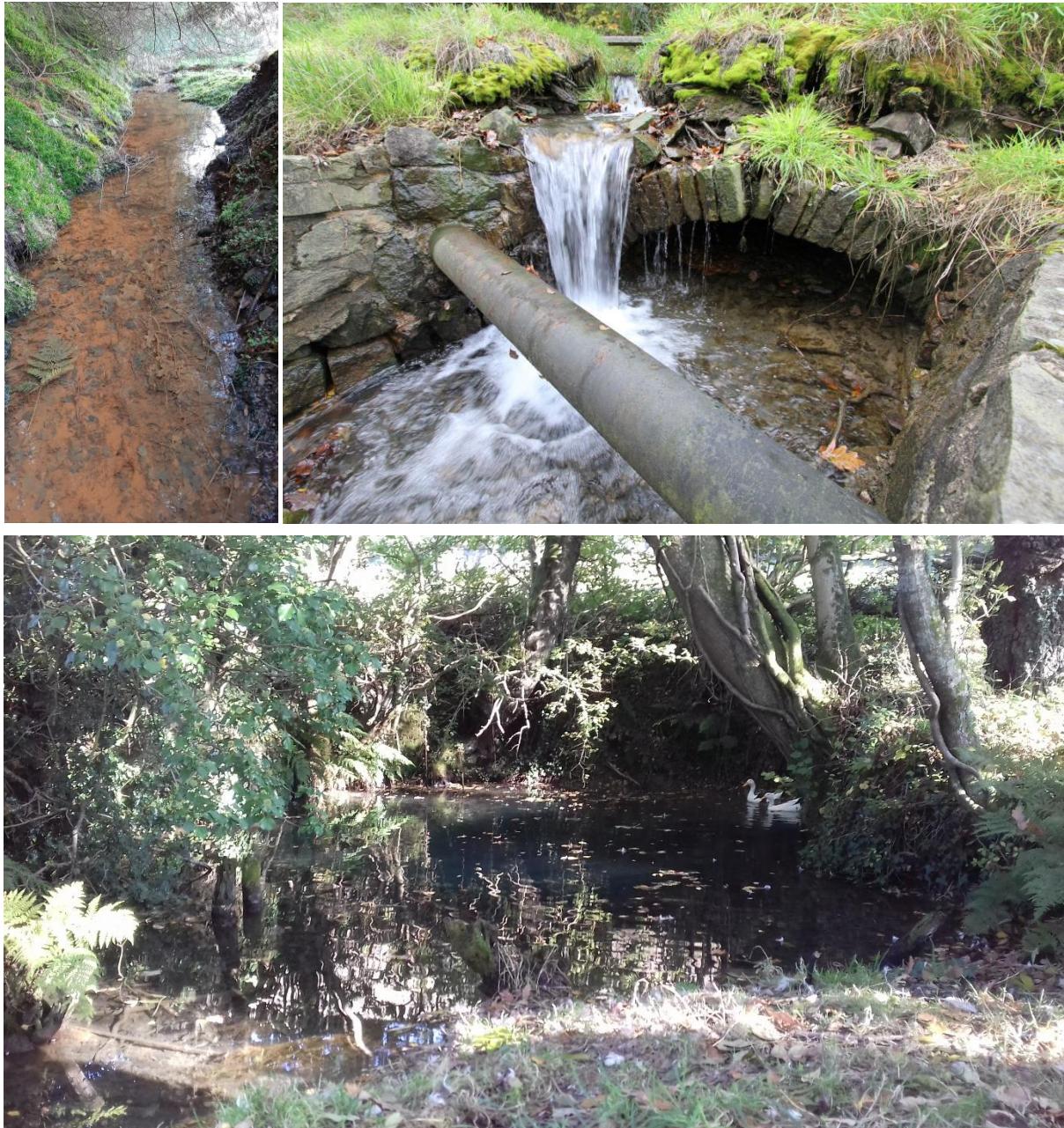
Figure 3-5 - The collapsed Upper Boat Level, top left, and crown of the blocked Deep Boat Level, top right (P. Edwards). The flow over the crown is from the flooded shaft in the lower photo.
