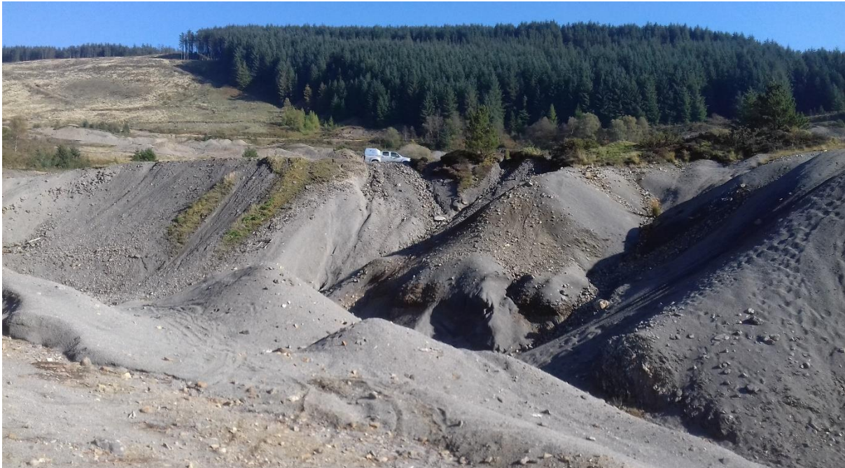
Figure 3-4 - the upper mine wastes at Nantymwyn, with NRW 4x4 for scale. Erosion to the mine wastes can be seen, from both surface water flow, and dirt bikers.
