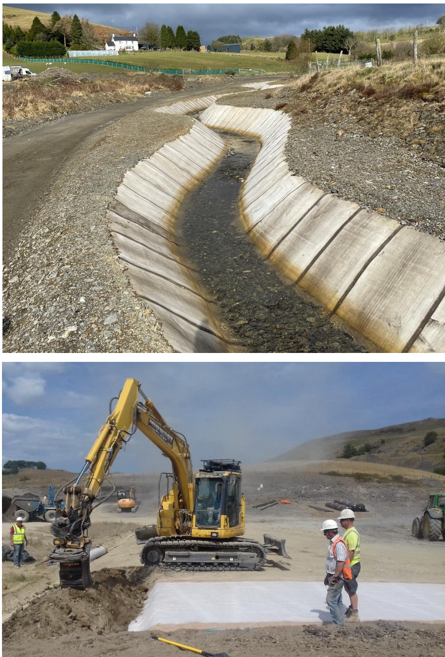
Figure 2-6 – Top, a lined and diverted stream at Frongoch lead zinc mine, mid Wales. Note mine wastes on either side of the stream. Bottom, capping the reprofiled mine wastes, with a geotechnical clay line (the white sheeting on the right) being covered with topsoil.
