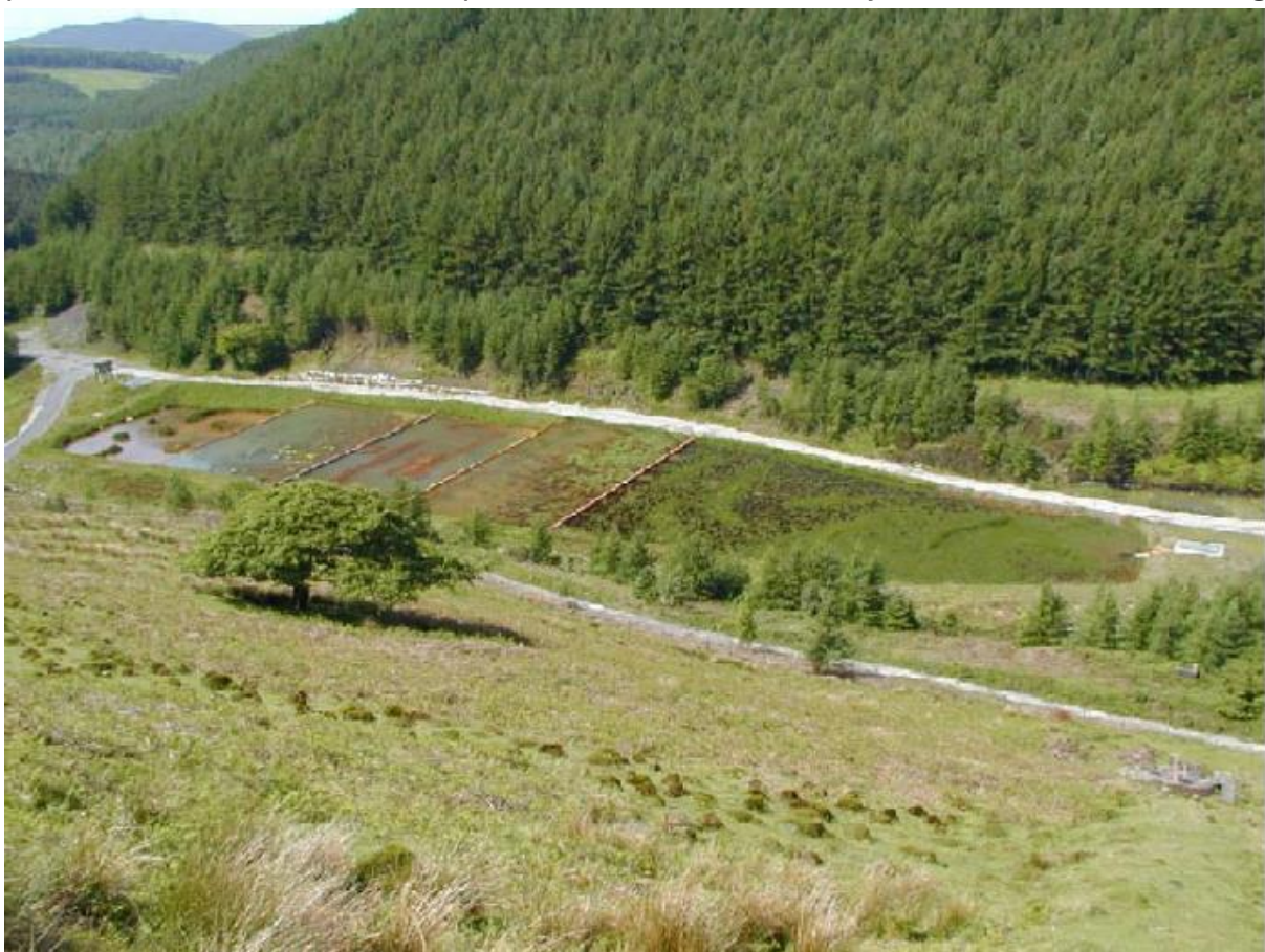
Figure 2-8 - one of the three passive minewater treatment systems at the abandoned Pelenna coal mine in South Wales. Minewater enters the system on the right and passes through it under gravity alone. Picture from (Wiseman et al. 2002).
