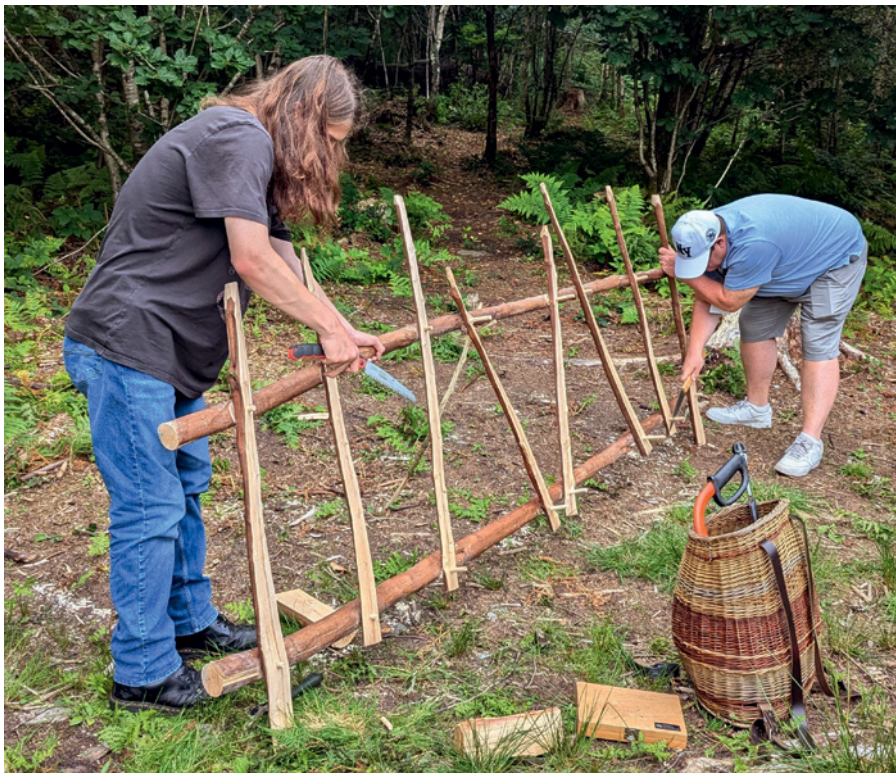
Photo 1. Wellbeing greenwood activities working towards hard fixtures and fittings for managing access at Craig Gwladus Country Park. Photo by Richard Manning.
