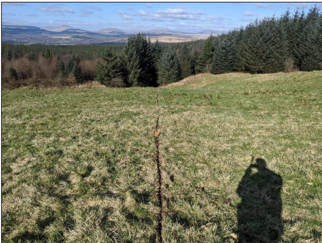
Figure 4.6: Photograph of trench cut using adapted lawn edger.
