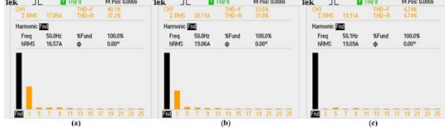
Fig. 10. Experimental harmonic spectrums of (a) load current, (b) grid current when only PPF is connected to PCC, (c) grid current when HAPF is also activated.
