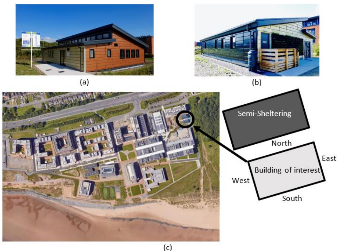
Figure 2. Building viewed from the (a) northwest, (b) southeast, and (c) location of the building and the façade names used for reference.
