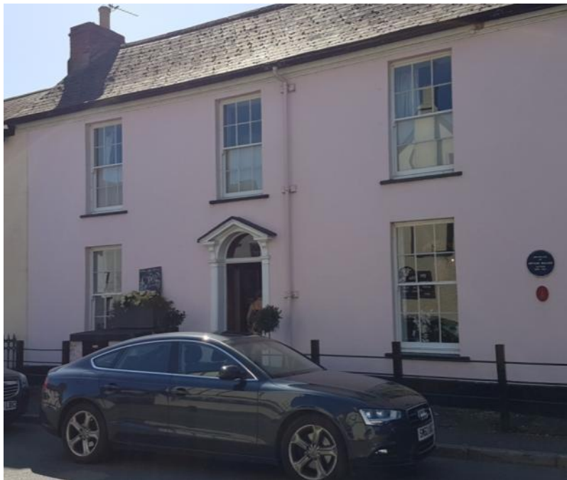
Figure 21 – Machen Interiors at 33 High Street, August 2019
