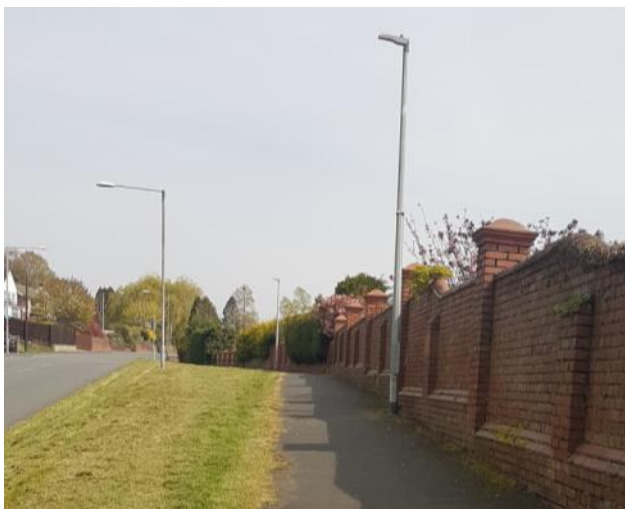
Figure 33 – Remnants of hospital wall, Lodge Road looking east, April 2019.
