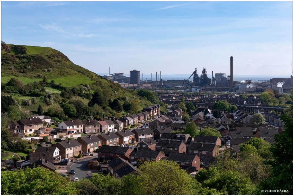
Figure 1.1: A view of Tata Steel Port Talbot as seen from the North. Pictured are the two operational blast furnaces, sinter plant, power plant and BOS plant (partially obscured). Images used with permission courtesy of Viktor Macha 8 .
