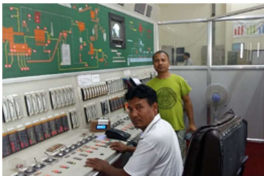
Control Room 2 UCIL with senior engineers Shaligram and Dan Bahadur
