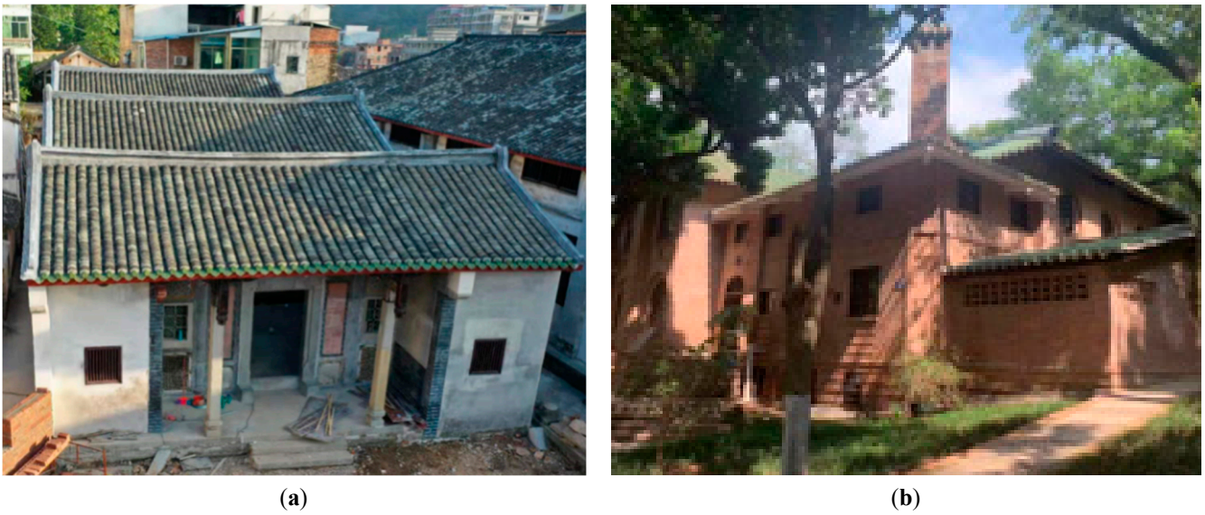
Figure 8. Historical sites for digital documentation in Guangdong, China: (a) Zou Lu House; (b) Wesley House.
