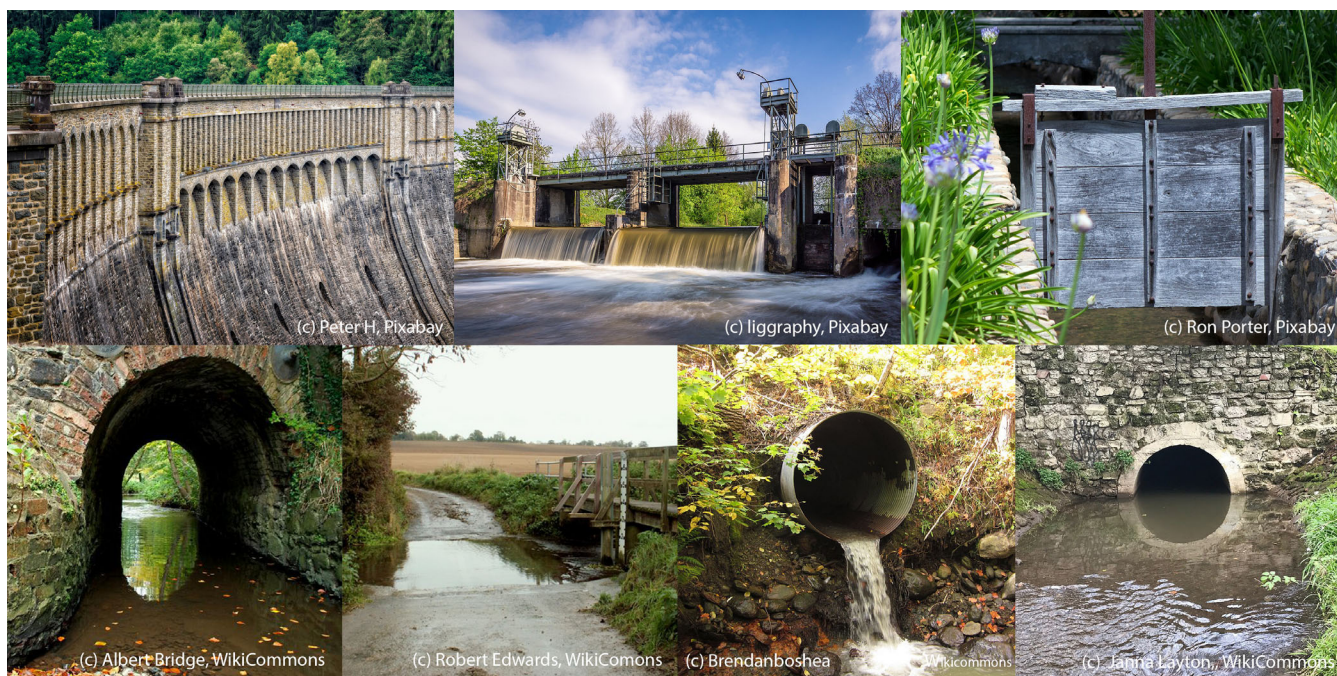
FIGURE 1 Examples of the instream infrastructure types (top row, L-R: dam, weir, sluice; bottom row L-R: bridge, ford, perched culvert, nonperched culvert) included in expert elicitation surveys about the passability of structures for elver European eels ( Anguilla anguilla ). Images were not provided to survey participants
