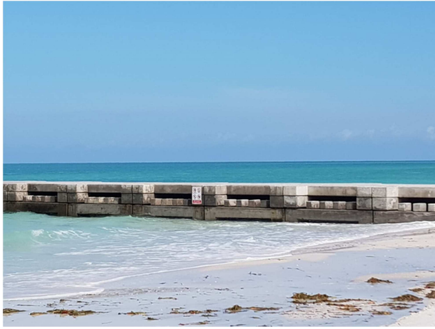
Fig. 19. The innovative groyne design concept that allows for adjustment of groyne permeability by adding/removing pre-cast concrete blocks (photo: Cortez beach, Florida).
