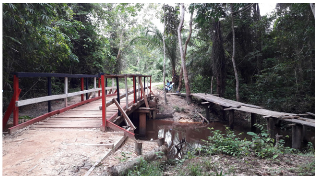
Figure 5. Newly constructed 'engineered timber bridge' (left) and old locally constructed bridge (right)
