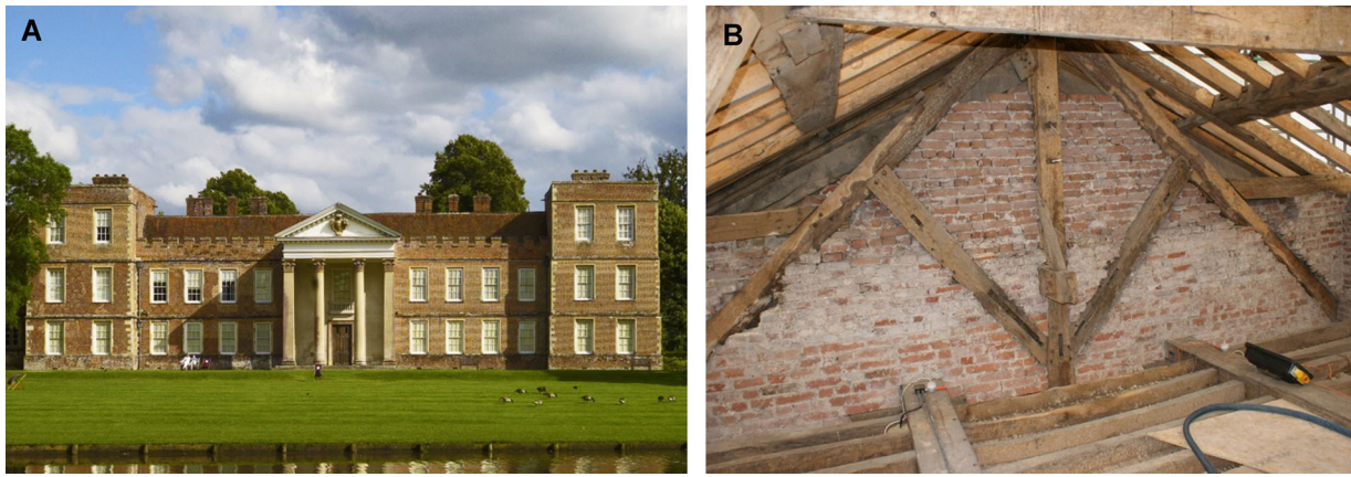
Figure 4. The Vyne Portico, Hampshire. (A) External view showing Webb's original portico, the first and oldest example on an English country house. (B) Internal view of portico showing sampled rafters. © The National Trust. [Color figure can be viewed at wileyonlinelibrary.com].
