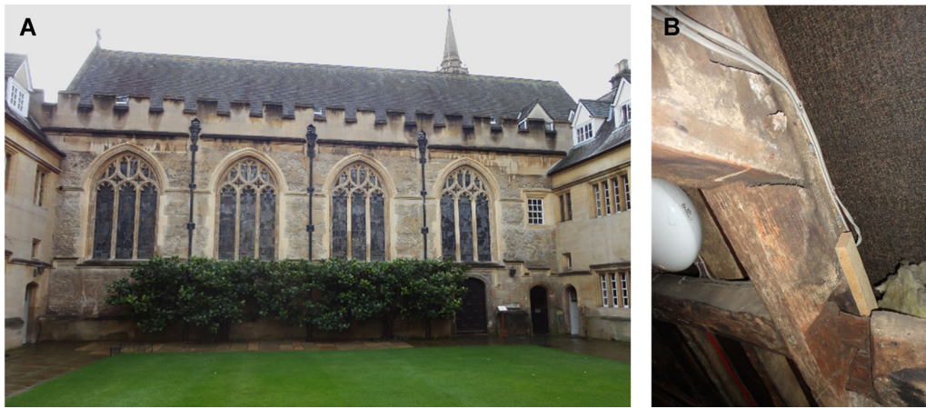
Figure 6. Lincoln College Chapel, Oxford. (A) External view. (B) Internal view of roof structure showing sampled rafters. © D. Miles. [Color figure can be viewed at wileyonlinelibrary.com ].
