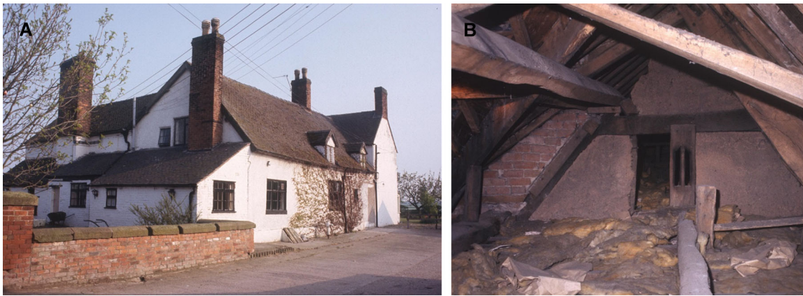
Figure 14. Oldfields Farm, Shropshire. (A) External view. (B) Internal view of roof structure showing king strut. © Madge Moran. [Color figure can be viewed at wileyonlinelibrary.com ].
