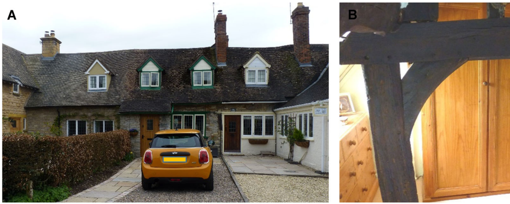
Figure 8. 2-6 Church Lane, Wilmcote, Warwickshire. (A) External view. (B) Internal view showing the head of a spere post. © N. Alcock. [Color figure can be viewed at wileyonlinelibrary.com].
