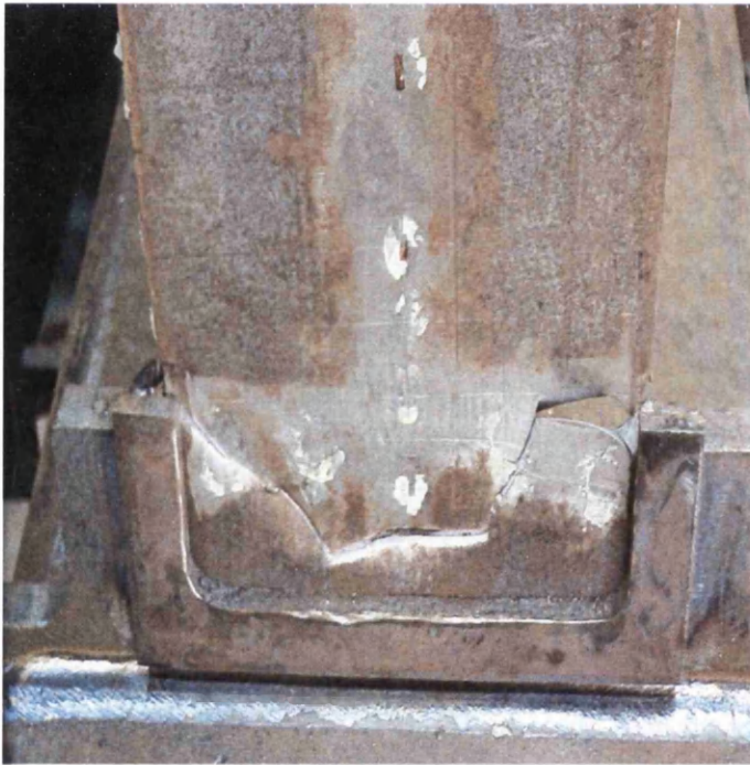
Figure 3.11 Tensile failure T-1 and 2
