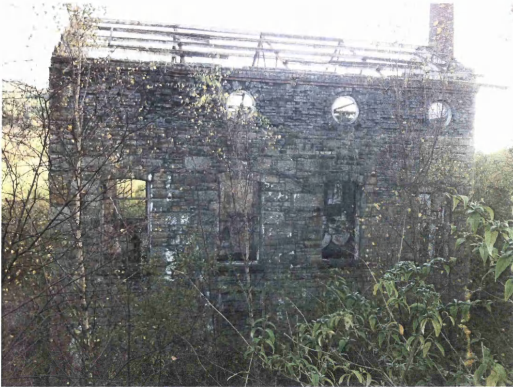
Figure 1.1: A crumbling building at the Hafod Copperworks (2012).
