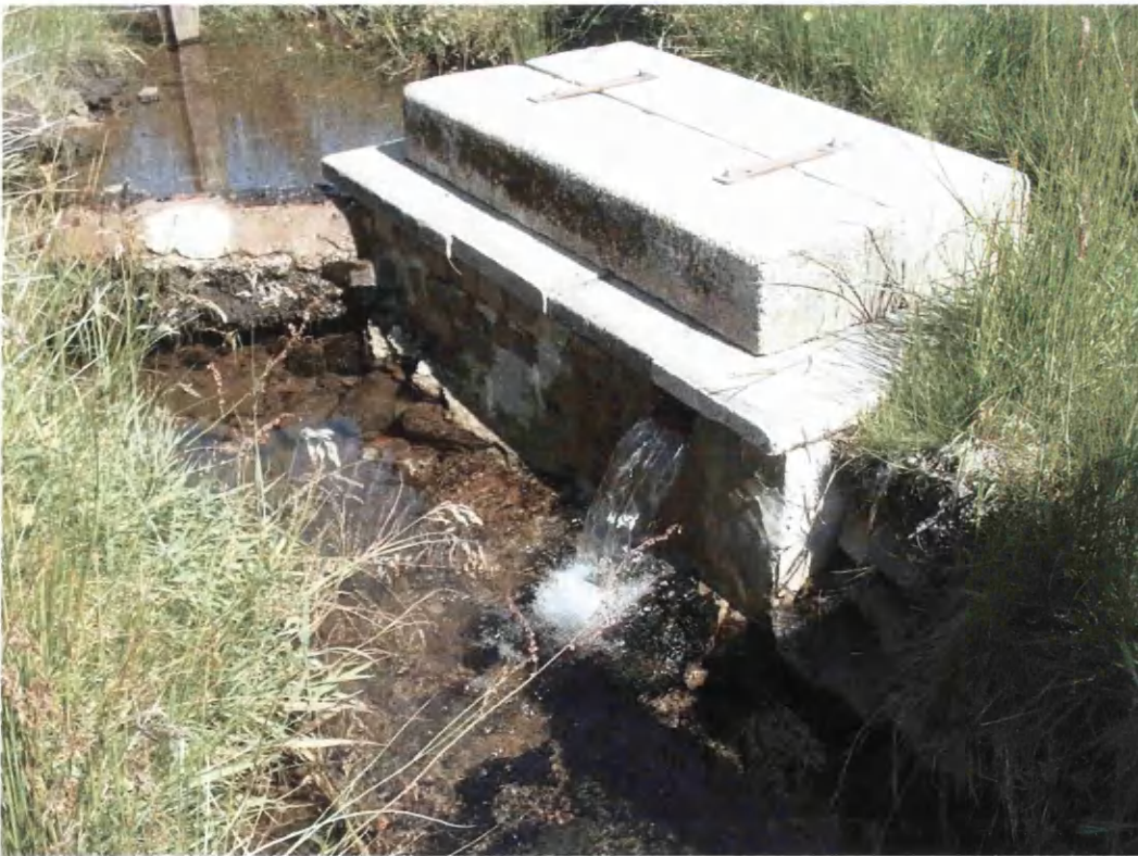
Picture 22: The abstraction point on the second burn, showing the off-take (with water over-spilling), and the weir regulating the water level
