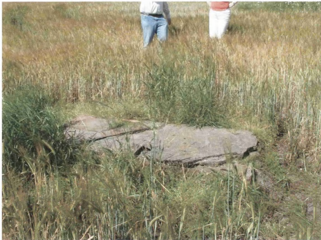
Picture 16: The settlement chamber, covered by a thick metal sheet, which is held in place by 3 broken stone slabs
