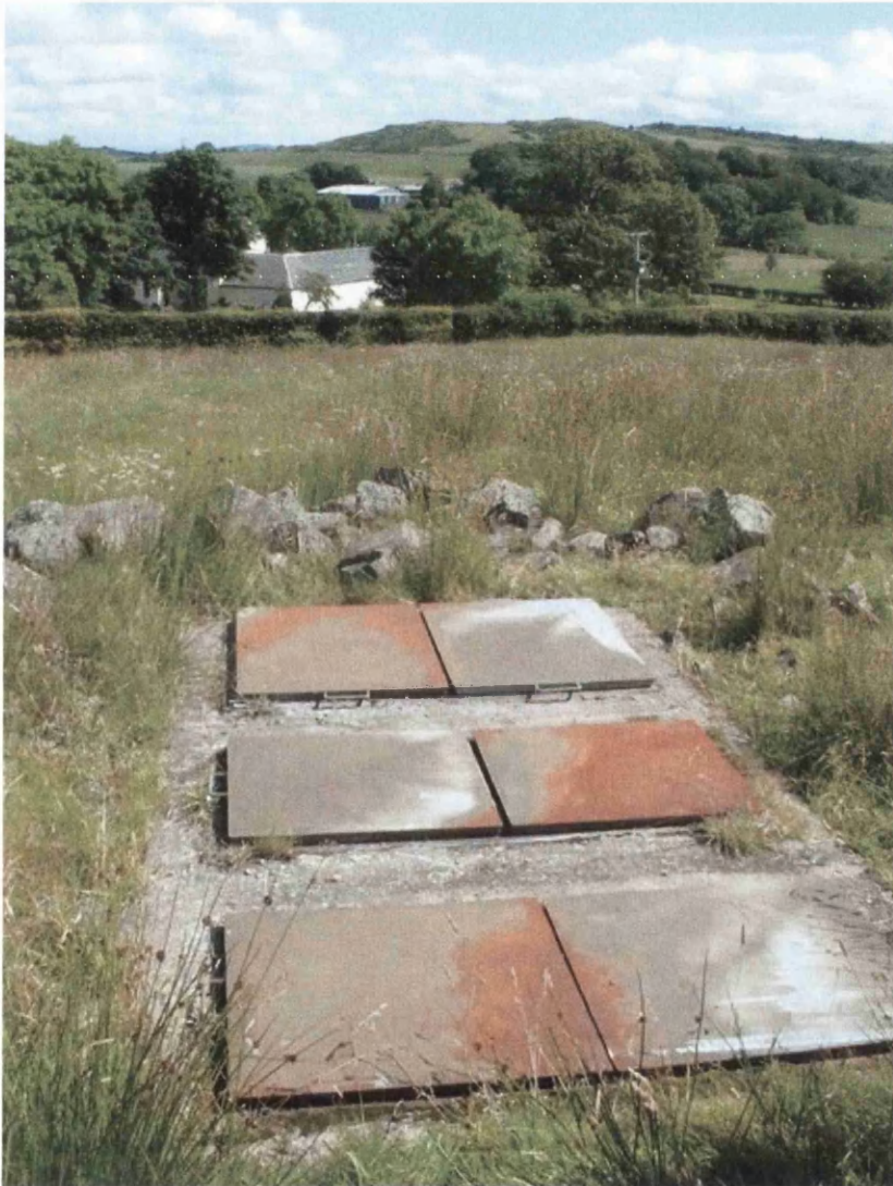
Picture 11: A view of the second collection chamber, consisting of three inter-connected settlement cells, looking east towards Farm '1'
