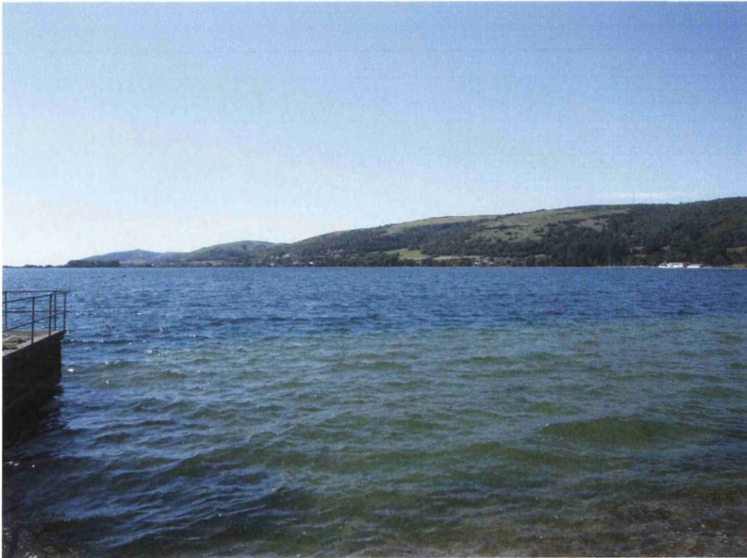
Picture 2: A general view of the reservoir, with the draw-off tower just visible in the left of the picture
