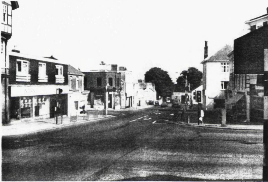
PLATE 6: KILLAY DISTRICT CENTRE
