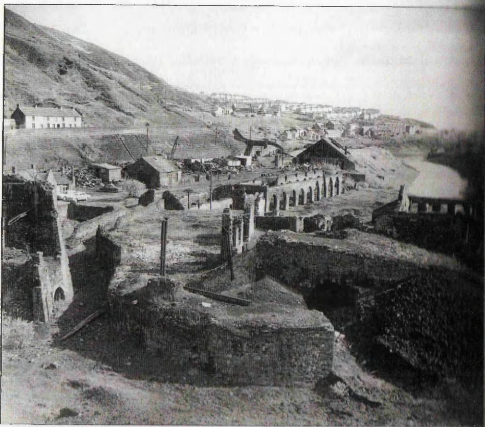
Ruins of the White Rock copperworks, before reclamation, Kilvey Hill is to the left, the river Tawe to the right. National Monuments Record for Wales.
