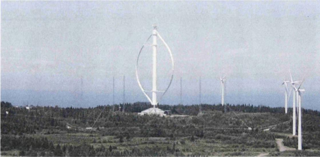
Figure 7.7: A Darrieus type wind turbine in Canada. Image by guillom-wikipedia.org.
