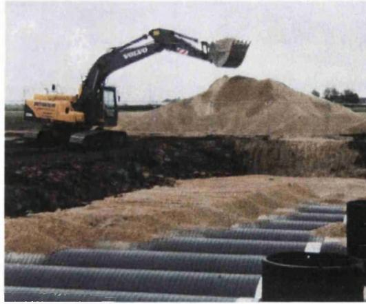
Figure 5.16: Additional installation loads induced by heavy machinery. This loading occurs after the installation is finalized for the particular area.
