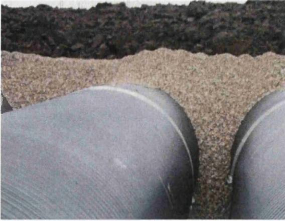
Figure 5.15: Illustration of installation soils. The primary backfill is a granular material and ends 0.3m above the pipe. The final backfill ends at the cover level and is a cohesive soil.
