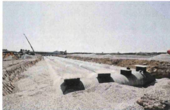
Figure 5.12: 1.8m diameter storage tank in Kent, UK.
