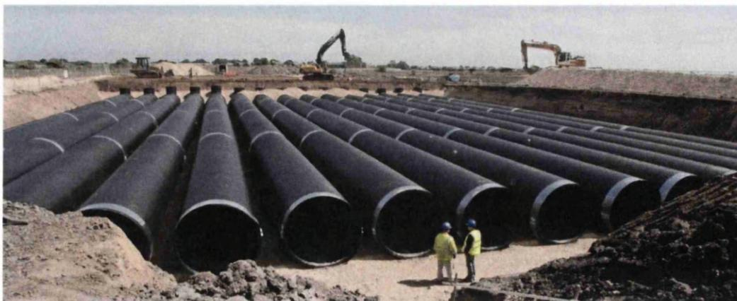
Figure 5.89: Construction site for the installation of 15 pipes prior to burying. The spacing between them is 0.5m, their diameter is 2.1m and the overall length of each leg is 114m.
