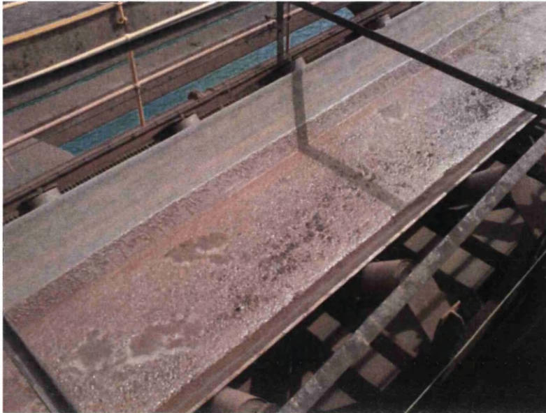
Figure 170: Fines ore saturated with moisture on harbour conveyor
