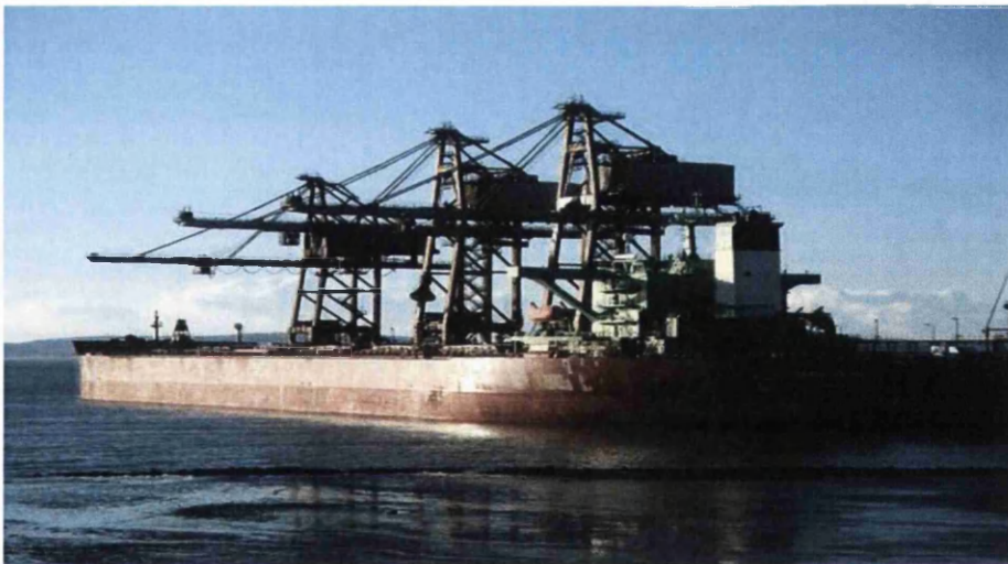
Figure 138: Three harbour ship unloaders working on the Berge Atlantic
