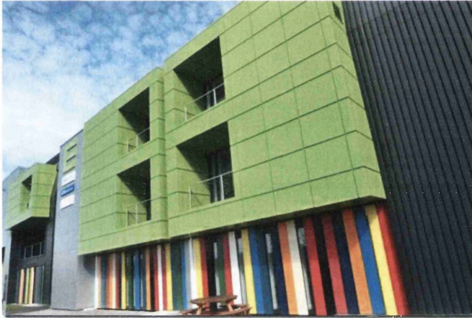
Figure 6.1 – Sustainable Building Envelope Centre, Tata Steel Incorporating a Range of Coloured Coil Coated Steel [1]
