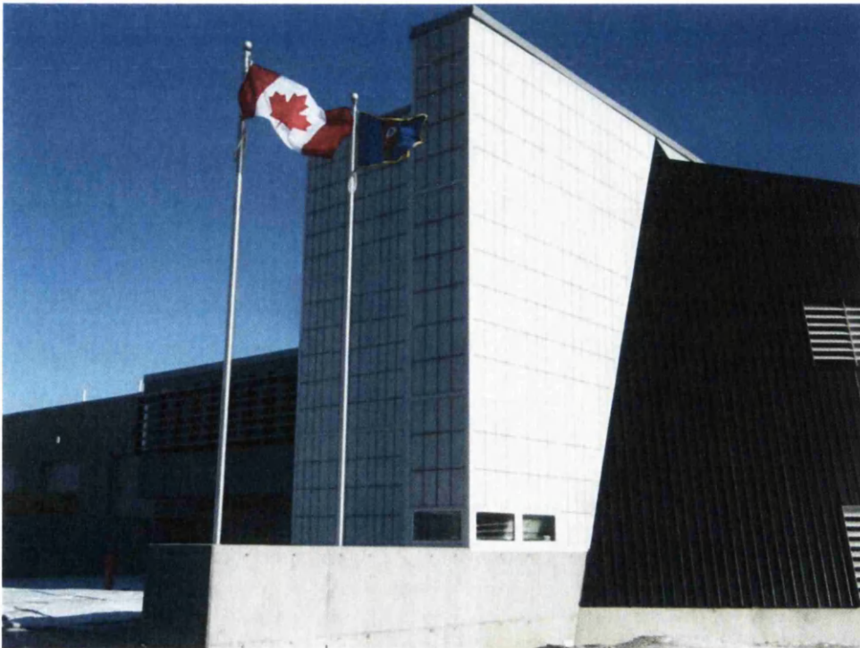
Figure 1.32 – Fire and Emergency Services Training Institute at Toronto Pearson International Airport, incorporating a Transpired Solar Collector Façade Image Copyright Conservat Engineering Inc. This work is licensed under the Creative Commons Attribution-Share Alike 3.0 Unported Licence.
