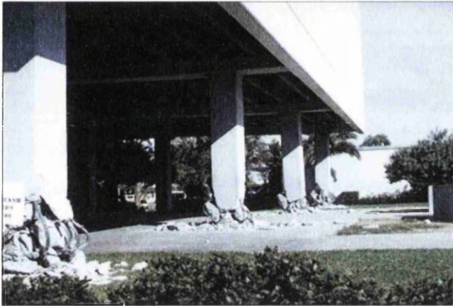
Figure 1.5 Destruction of plastic hinge zones [5]
