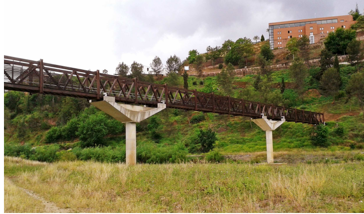
(a) Montoro bridge over the Guadalquivir river
