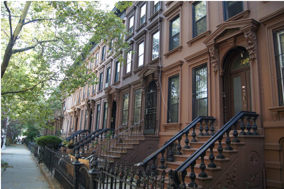
Fig. 9 Brownstones in Fort Greene. These brownstones have four stories. It is not uncommon to have more than one apartment in each floor. Source: Photo taken by the author, 2014
